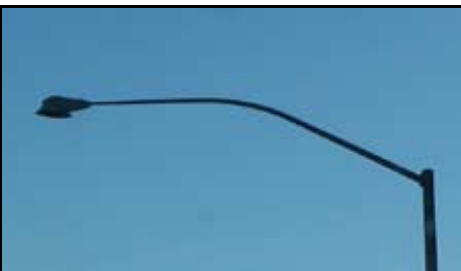
An example of full cut-off lighting used in Flagstaff, Arizona. Flagstaff is roughly the same size as Peterborough, yet one can easily see the Milky-Way, even in town.
